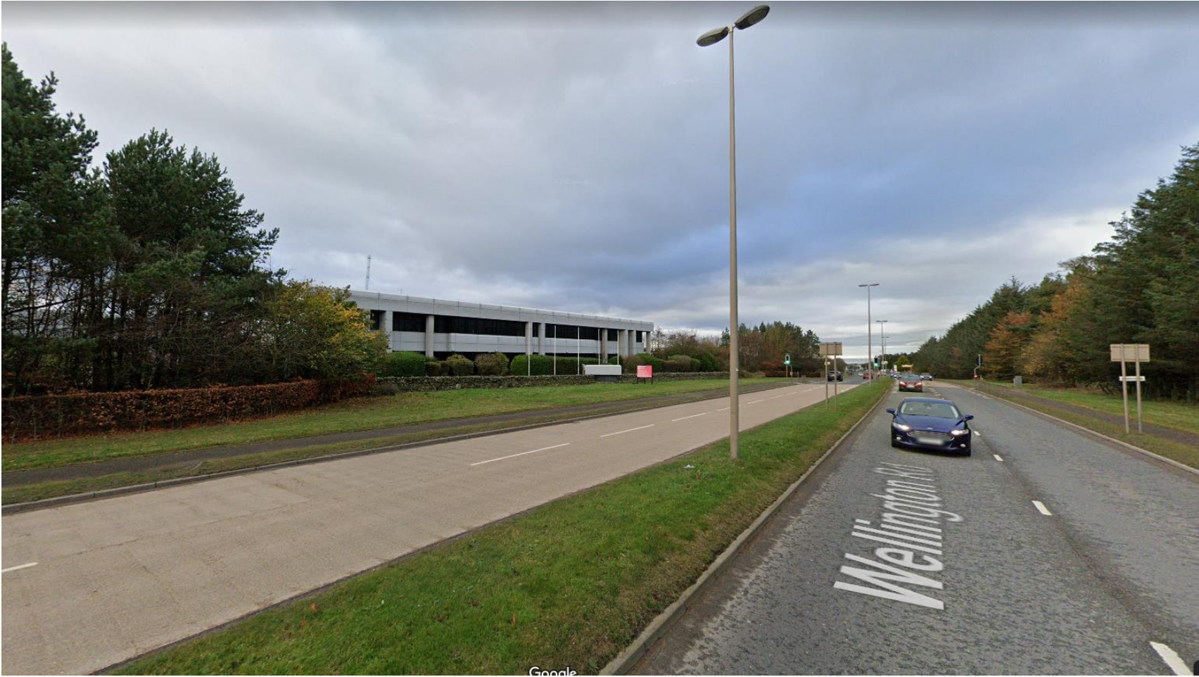
Looking north from Wellington Road
